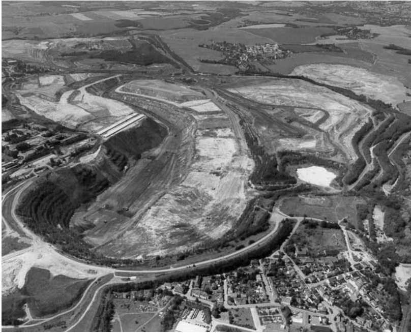
Fig. 6: Backfilling of the worked-out open pit mine
