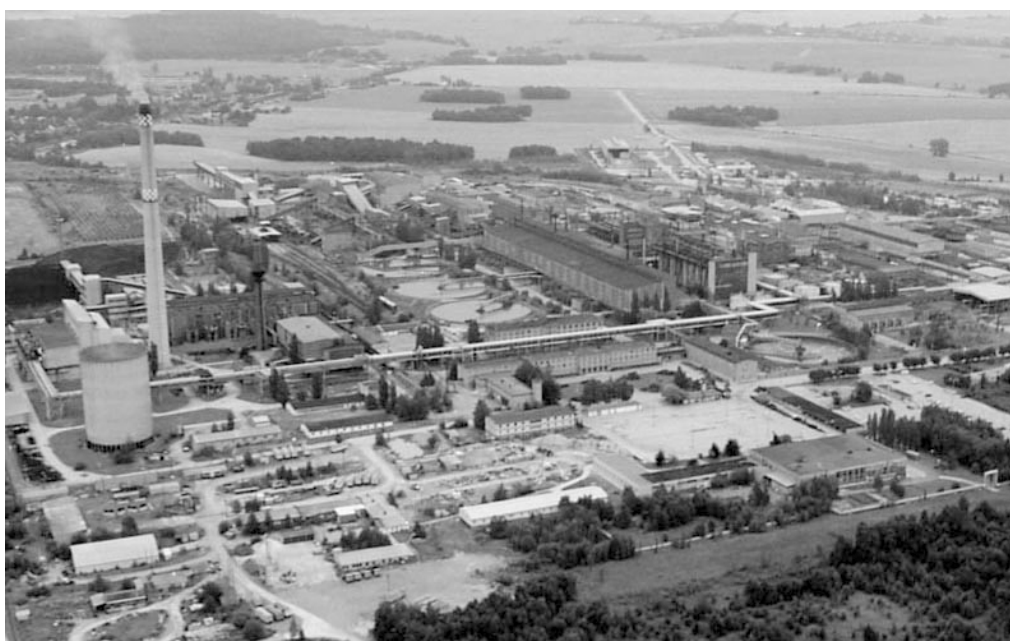
Fig. 3: Former uranium ore processing plant at Seelingstädt in Thuringia, East Germany (photo shot in 1991, the facility has been demolished and the site reclaimed)
