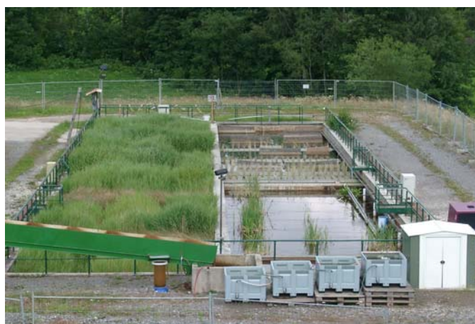
Figure 4 View of the pilot wetland, the aeration cascade is visible in the left lower corner. In the foreground, there are plastic ponds used for Radium sorption tests with algae.
