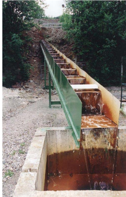
Figure 5 Aeration cascade between the mine adit and the inflow to the pilot wetland. The dark stain from iron precipitates is clearly visible.
