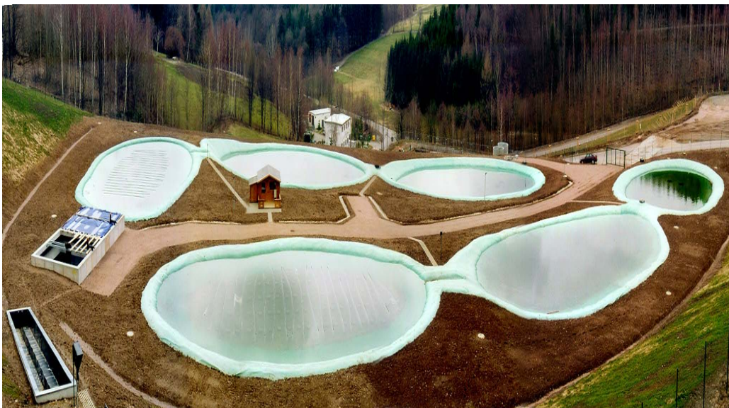
Figure 9 Aerial view of the full scale wetland at the Pöhla site. The double-line structure can be clearly seen, with one line in the upper part of the photograph and the second line in the lower. In the left lower corner, the aeration cascade is visible, followed by the rectangular settlement pond (concrete structure).
